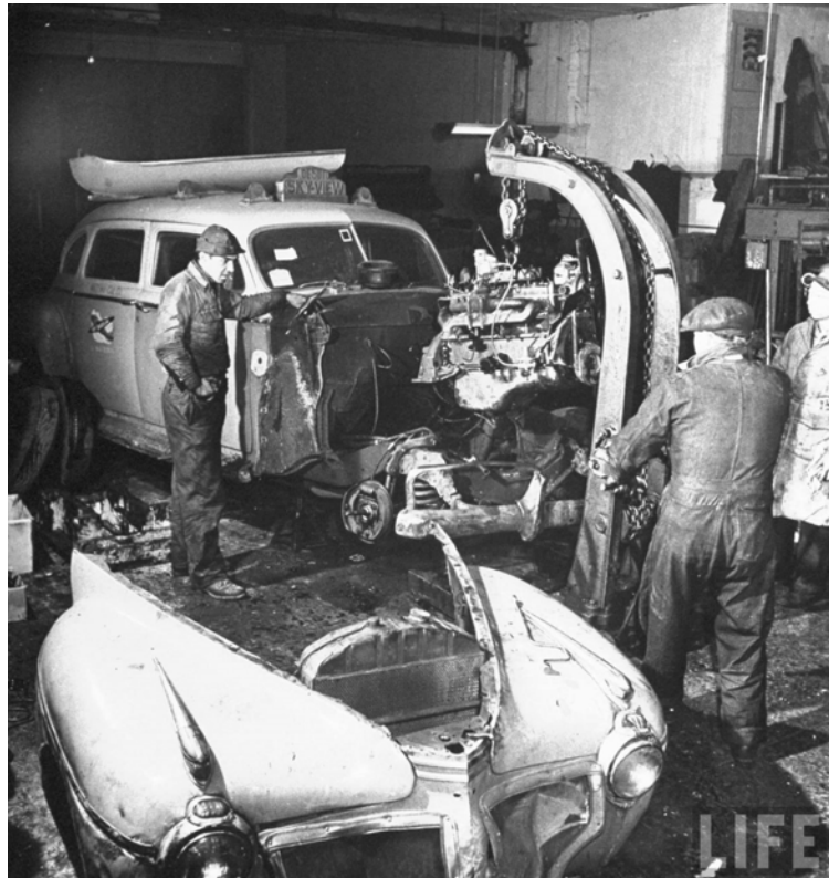
Auto mechanics using hoist to drop in motor of taxicab under repair at company's maintenance garage
